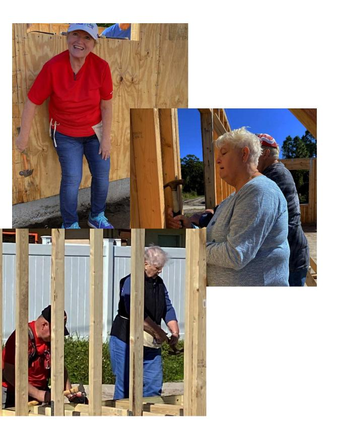
In 2021 we started with a bare, concrete slab and piles of 2x4 lumber. We worked from 0730 to 1200 hrs – half days – for two days working side-by-side with the future homeowner, and the very patient Habitat construction supervisors. When our time was up all four walls were up and covered – quite an accomplishment!
